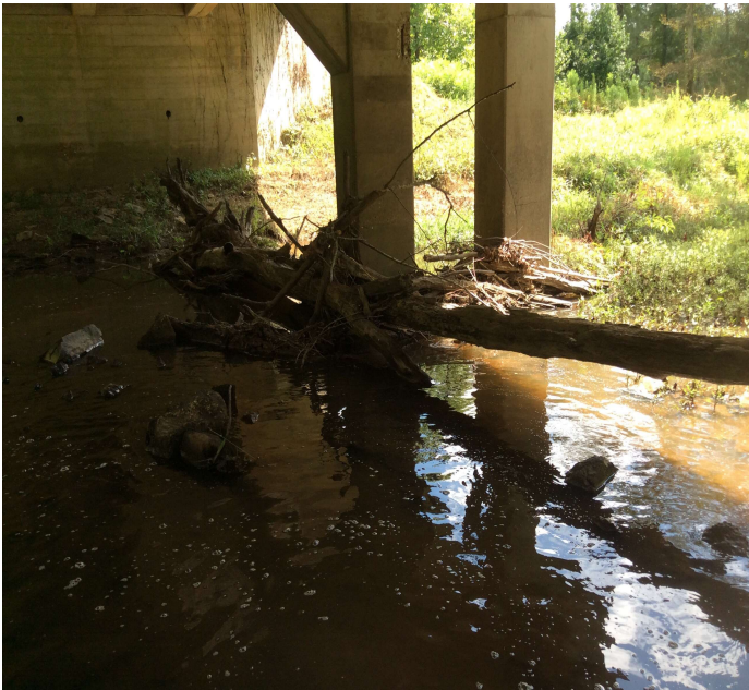
PHOTO 1 Description Drift built up on column 3 at Bt. 2.
